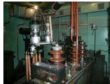
2 nd Klystron Supply
