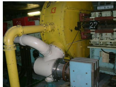
Titanium Vacuum Pumps
